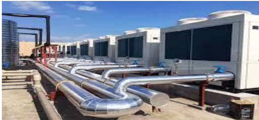
Chilled Water / Hot Water Line fabrication and Thermo Insulation works
