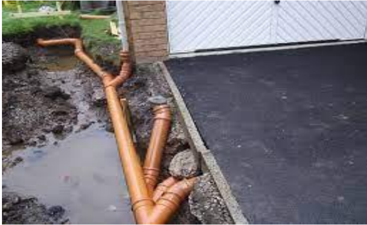
Plumbing and Drainage Lines works
