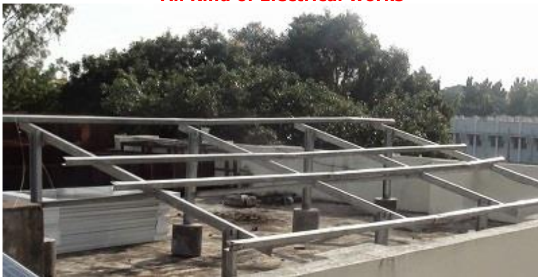
Solar Panel Structural Works
