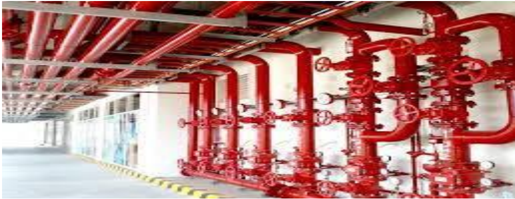
Fire Fighting Hydrant and Sprinkler line Fabrication and Repairs
