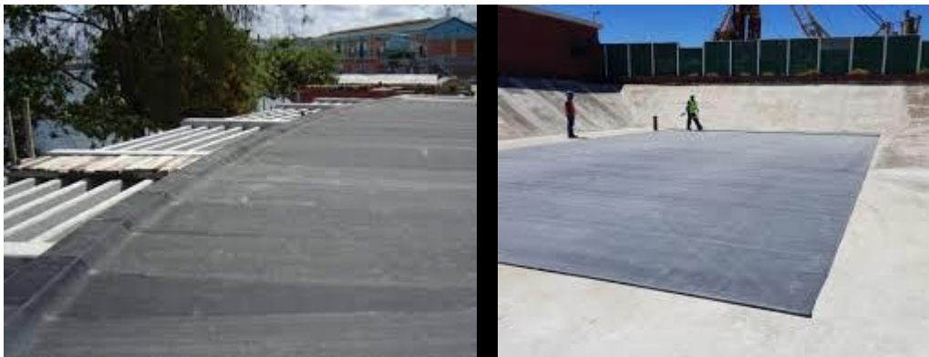
Membrane and Synthetic Water proofing works
