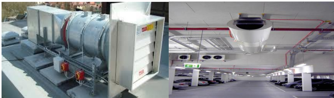
Staircase Pressurization system and Smoke Extraction System Fabrication and installation
